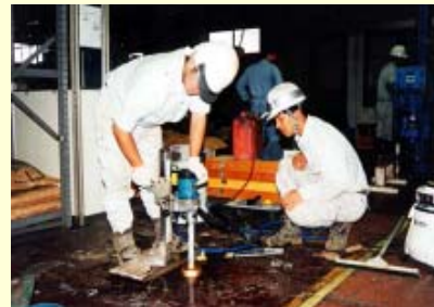
Investigating the soil on the premises
