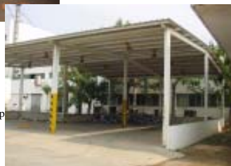
Oil retaining floor at iron scrap shed to prevent soil pollution from machine oil contained in iron scrap (Dalian Mabuchi)
