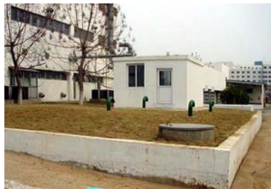
Spring water utility in Dalian Mabuchi (Dalian City, China)
