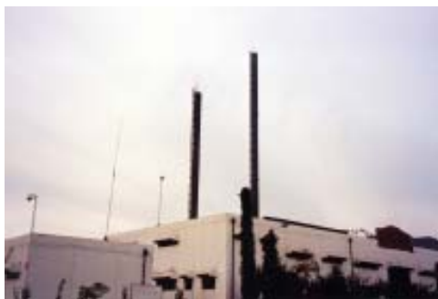
Dalian Mabuchi boiler room, introducing the energy-saving boiler and the latest model of dust collector with desulfurizer
