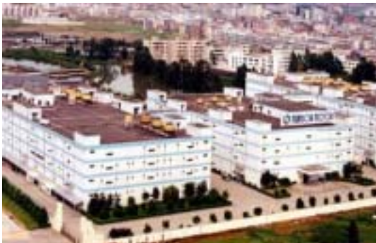
Mabuchi Motor is constructing new factories always keeping energy saving in mind. This picture shows a new office building of Guangdong Mabuchi Factory 1. Mabuchi Motor has introduced many energy-saving technologies in this building.
