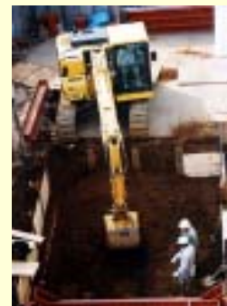
Excavating the polluted soil
