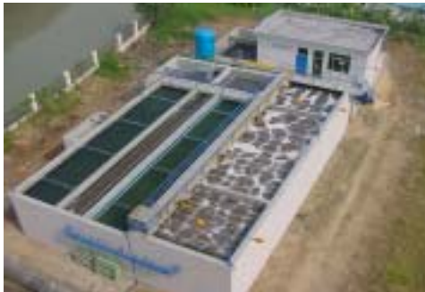
Sewage utility built in Factory 1, Guangdong Mabuchi
