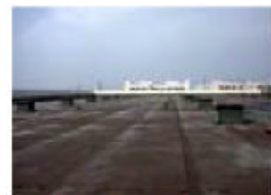
Before modification work
