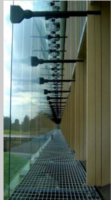
Above: Air-conditioning burden is reduced by promoting heat exhaust through the chimney effect created by the structure's double skin as well as by natural ventilation in conjunction with the atrium's skylight at dusk and at night.
