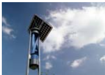
Streetlights powered by solar and wind energy
