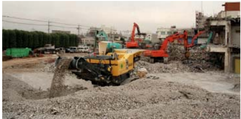
Crushing and sorting of demolition debris
