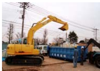
Demolition debris being shipped for recycling
