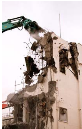
Demolishing the old office building
