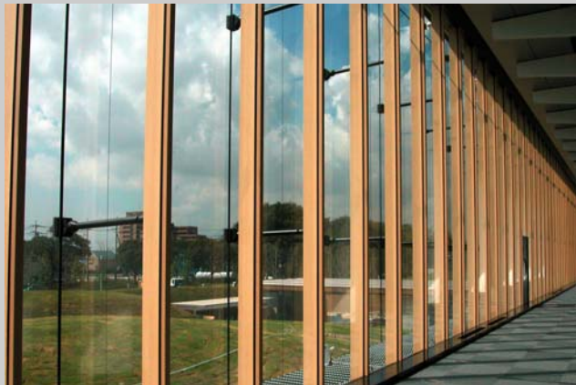
Above: Air-conditioning burden is reduced by promoting heat exhaust through the chimney effect created by the structure's double skin as well as by natural ventilation in conjunction with the atrium's skylight at dusk and at night.
