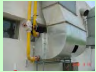
Air intake of an absorption type air-conditioner in the Dalian Mabuchi factory
