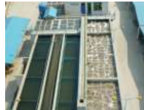
Wastewater purification and treatment facility
