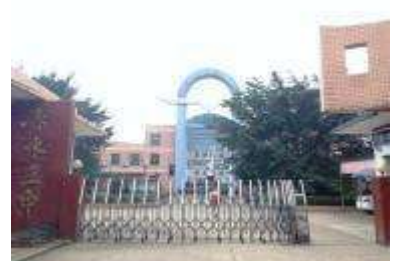
Support for constructing computer rooms in junior high schools (Daojiao Mabuchi)
