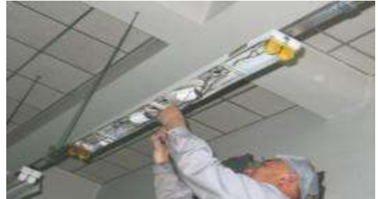
Replacement of fluorescent lights with LED ones (Dalian Mabuchi)
