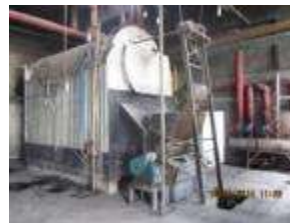
Boiler room before installing the central heating system (Wafangdian Mabuchi)
