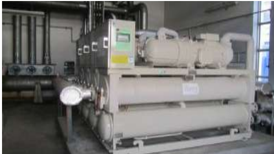
New chiller (Dalian and Wafangdian Mabuchi)
