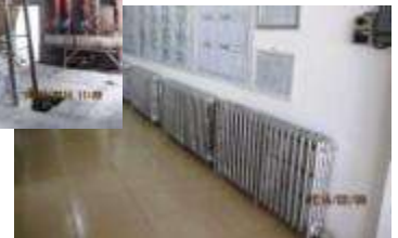
Inside the factory after installing the central heating system
