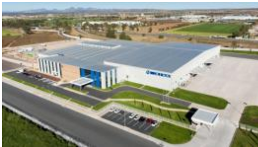
Construction of a new factory (Mexico)
